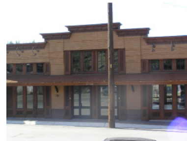
Flat roof lines
