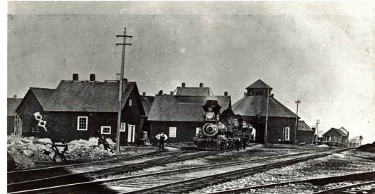
1875: A larger roundtable was constructed, tracks were raised to allow for easier snow removal and a large woodshed was constructed along the tracks to house the wood to fuel the trains.
